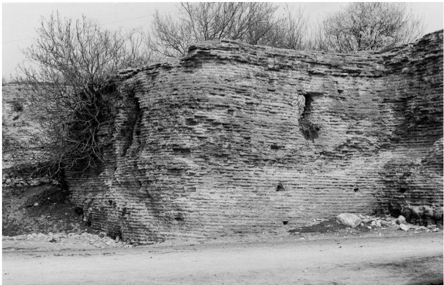
Figure 6: The North gate tower at Midye/Kiyiköy (Salmydessos). Like the late phase at Sofia (Serdica) the defences are constructed solely in brick, now restored. Credits/sources: Crow.
